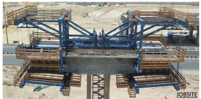
ABOVE, MIDDLE AND FAR RIGHT: The virtual formwork planning of the cantilever forming traveller (CFT) system using the DokaCAD for Revit software supported project implementation on the actual construction site.
