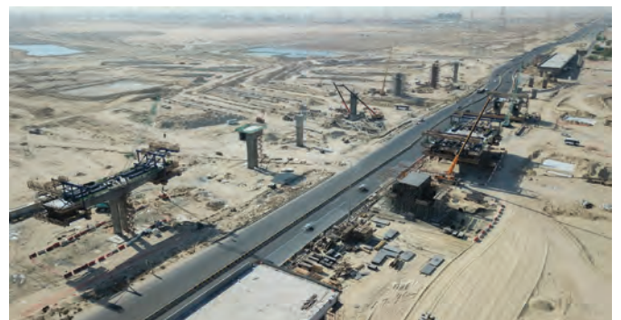
TOP AND ABOVE: Nawaseeb Road is an important element of Kuwait's transport infrastructure. The bridge project is a special case for two reasons: not only is it currently the country's first cantilever bridge project, but it is also the first time a bridge is cast in-situ.
