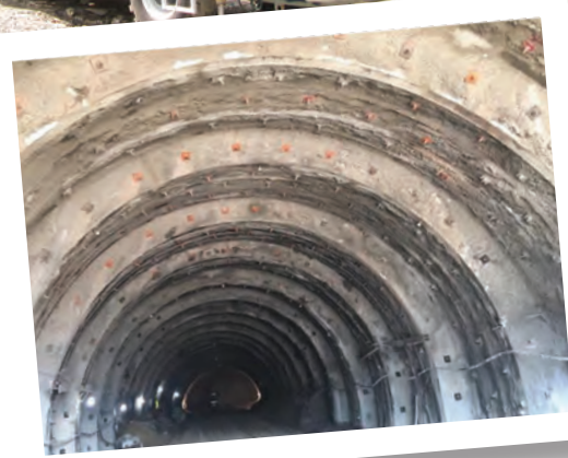
Mapei admixtures were chosen for this project. Two of them were used to produce shotcrete - which was sprayed on the tunnel walls (top and above) - and the other two for the tunnel linings (right).
