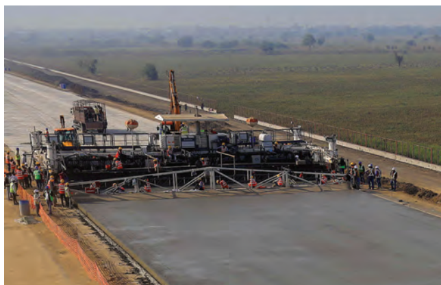
ABOVE AND LEFT: Local construction company Patel Infrastructure has set some new world records with the help of a Wirtgen SP 1600 slipform paver.
