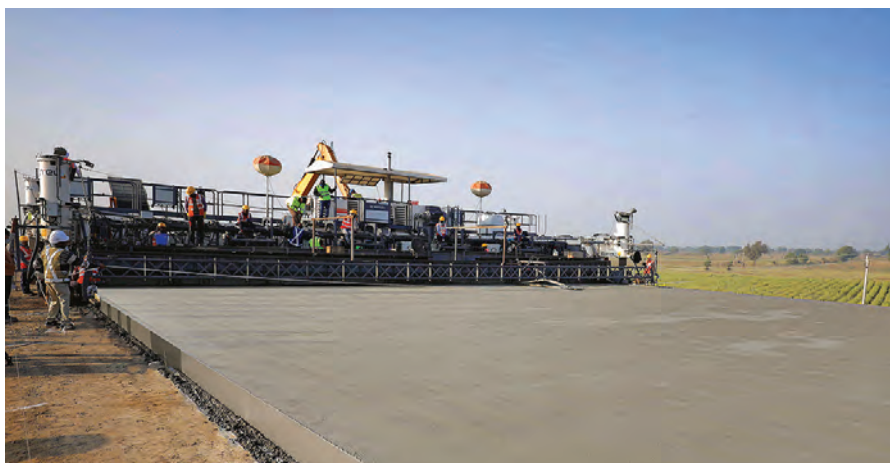
ABOVE AND LEFT: Local construction company Patel Infrastructure has set some new world records with the help of a Wirtgen SP 1600 slipform paver.
