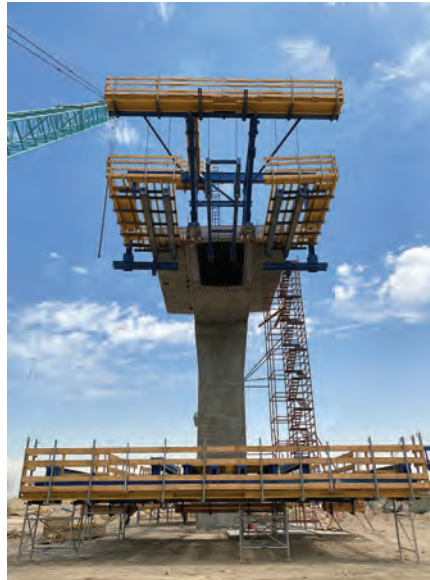
ABOVE, MIDDLE AND FAR RIGHT: The virtual formwork planning of the cantilever forming traveller (CFT) system using the DokaCAD for Revit software supported project implementation on the actual construction site.
