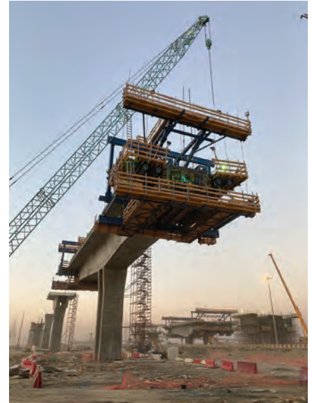
ABOVE, MIDDLE AND FAR RIGHT: The virtual formwork planning of the cantilever forming traveller (CFT) system using the DokaCAD for Revit software supported project implementation on the actual construction site.
