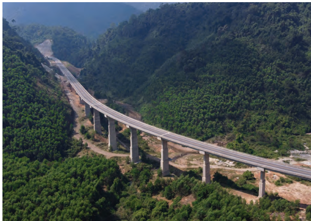
The Mui Trau twin tunnels in the Hoa Vang District (top), each featuring 2,260 m long, are part of the new La Son-Tuy Loan Expressway (above).
